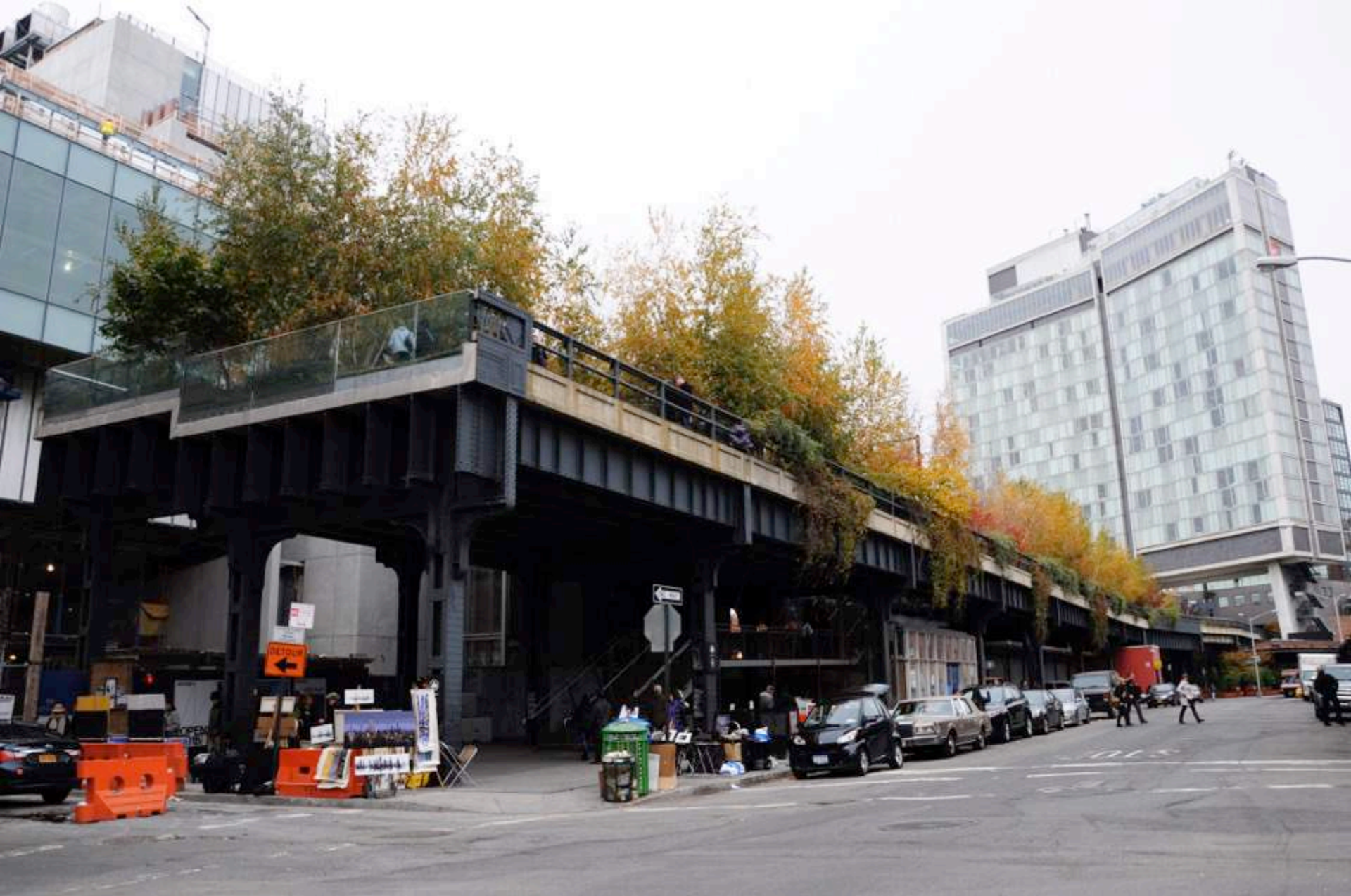
The High Line, James Corner Field Operation, Diller Scofidio + Renfro, New York, 2007-2016
